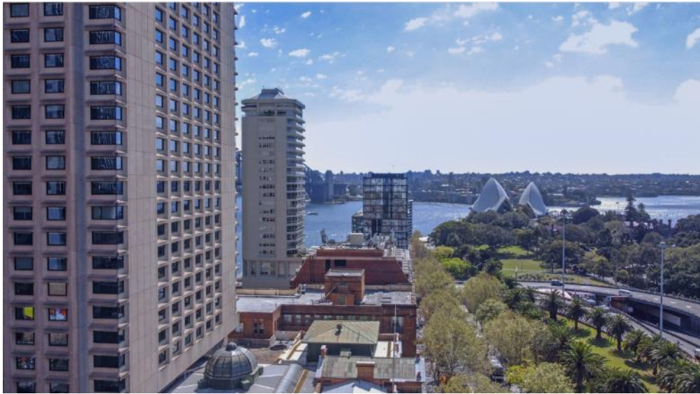
Figure 40: Drone photo from northern elevation of the Astor building facing north
